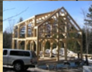
A timber frame home in Dublin; the entire frame was milled from trees cut directly from the cli- ent's property.
